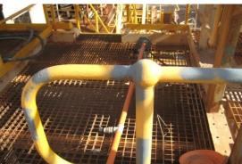
Figure 4.2 Mild Surface Corrosion & Remedial Treatment
