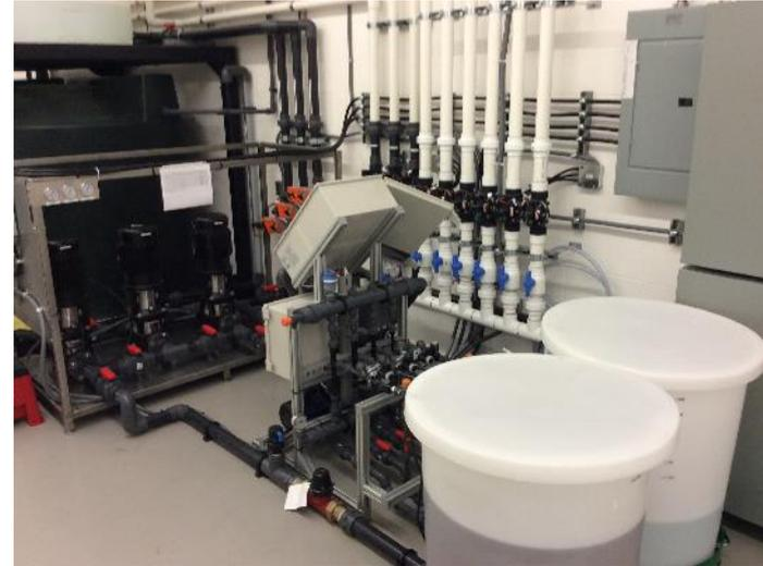
**Figure 2: Duncan Facility automated fertilizer system.**
