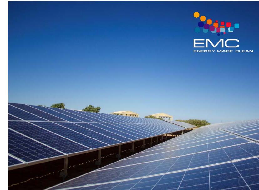
Remote monitored and controlled 100 kW PV /110 kVA Diesel/ 64 kWh battery project in outback Australia
