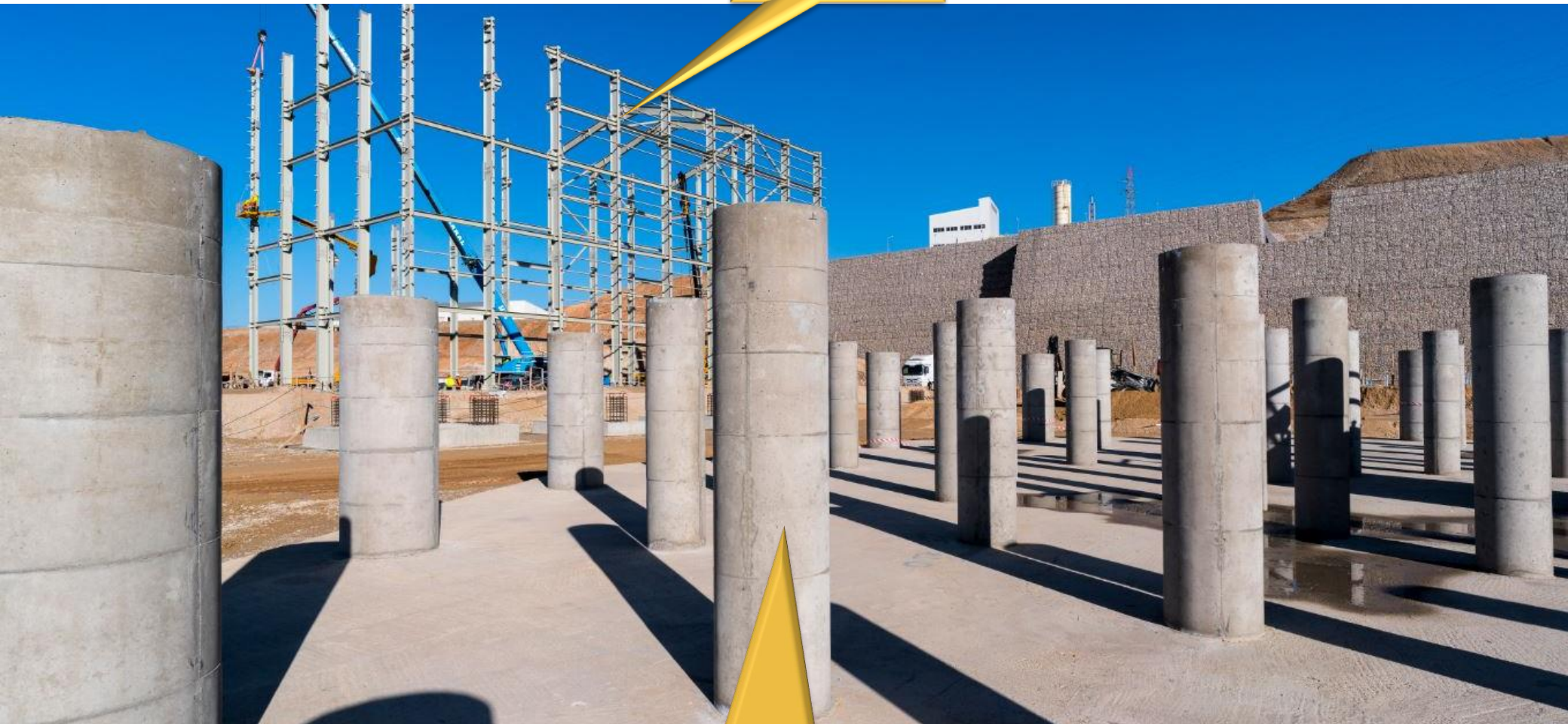
Decant Thickener Pedestals
