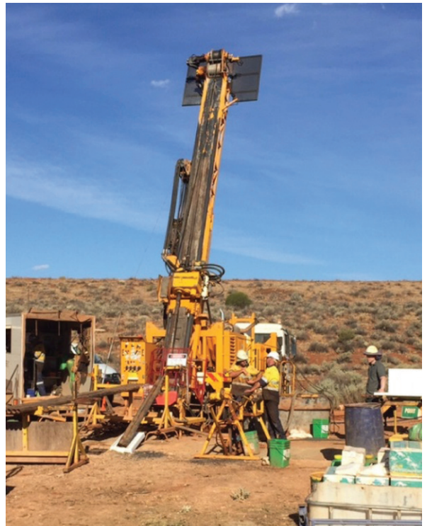
Drilling in progress at Nambi Prospect
