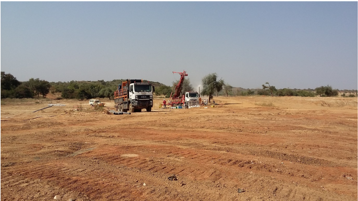
Before and after photos: M1 South - Sections SE425 to SE475
