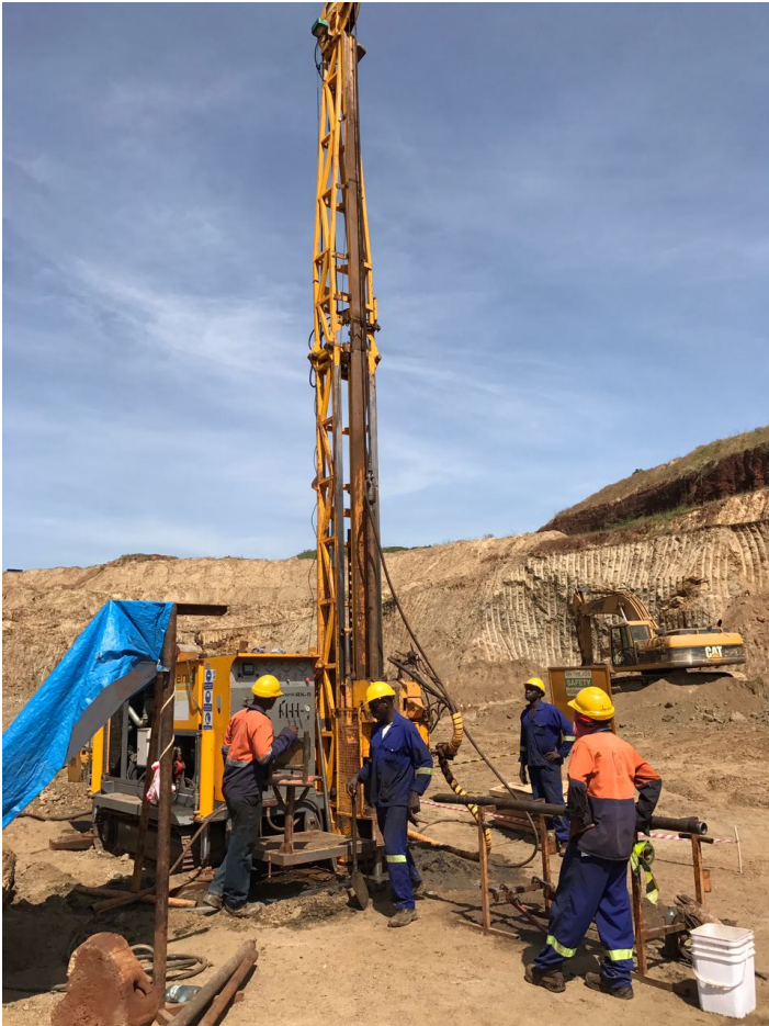
Fig 1. Air core drilling in P1 -the current open pit
