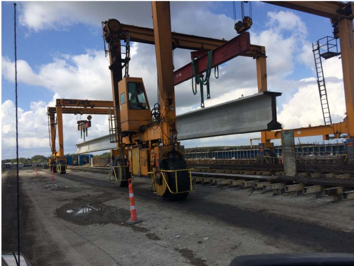
Figure 1. Typical Precast / prestressed bridge beam being fabricated
