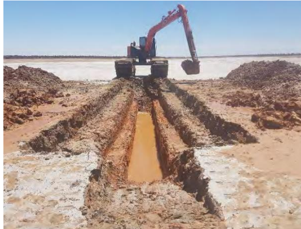
Photo: Trench excavation at Lake Wells 1 Significant trenching required to access low grade brines
