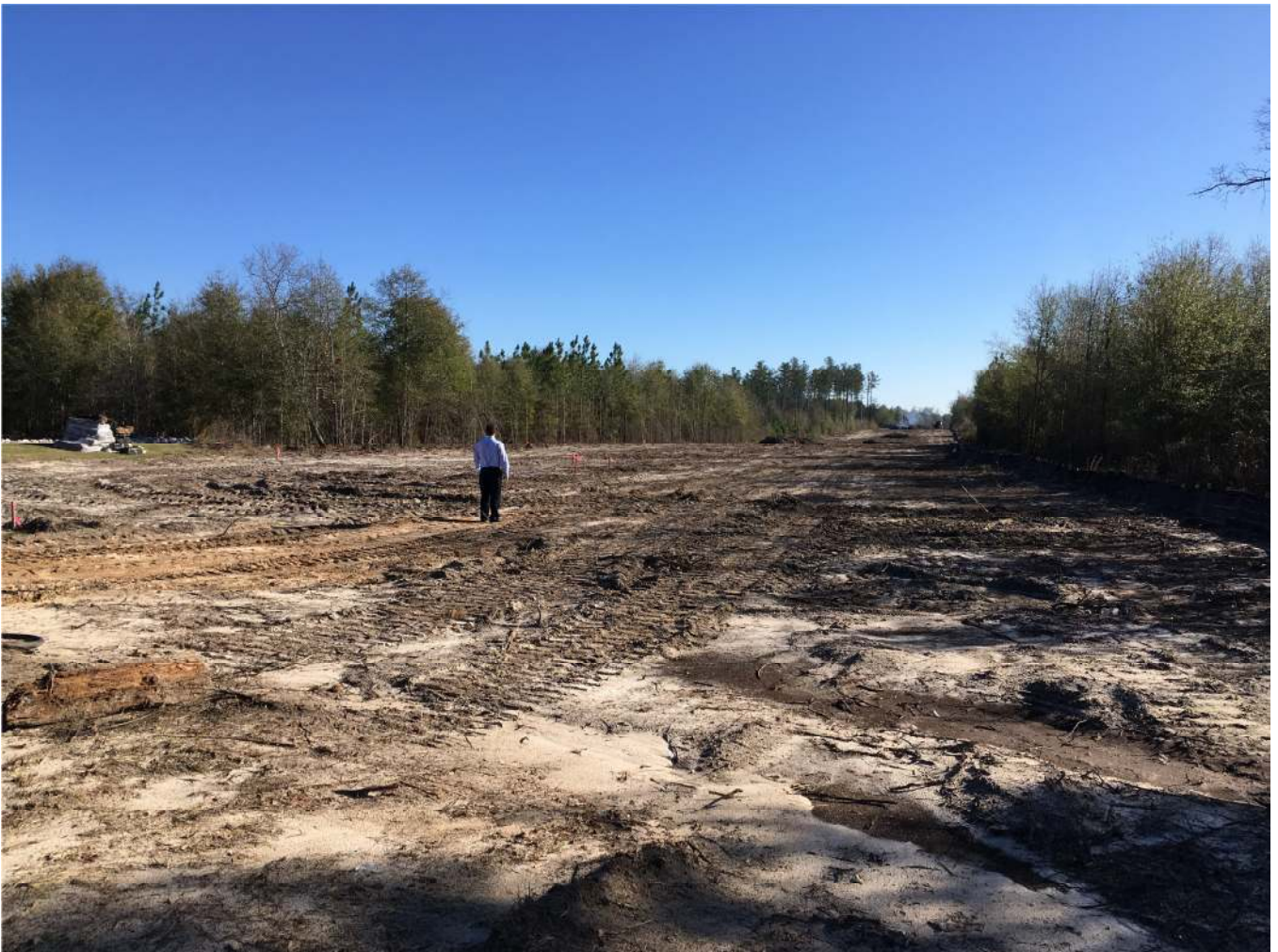
Figure 3. Clearing new access road to Proposed Augusta plant
