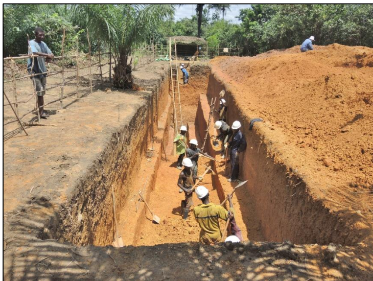
Figure 16. Excavation of trench (at left), over probe-positive KIM soil-sampling results obtained for the AM Geophysical anomaly, POD 011, EL 11/2014. The causative magnetic body proved to be a diabase dyke (at right). The source of the KIM ilmenites is unresolved.
