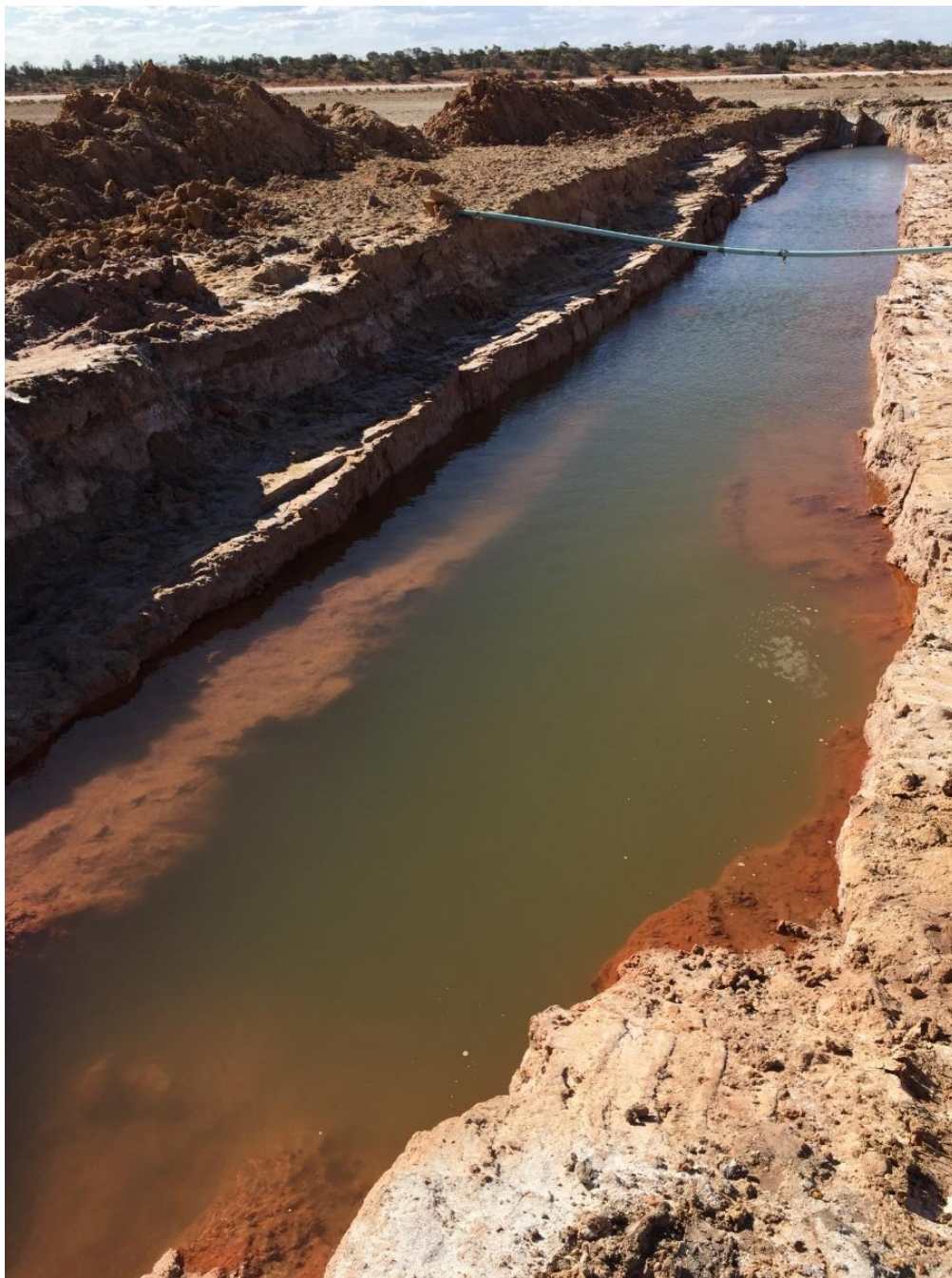
Figure 5: Trench P1c at Lake Wells
