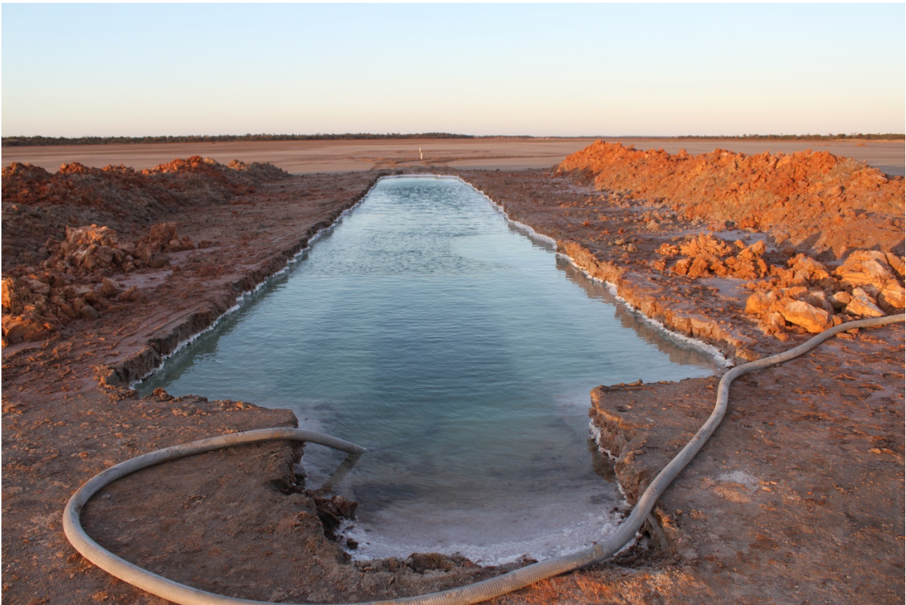
Figure 4: Trench Pump Testing in Progress at Trench P1a
