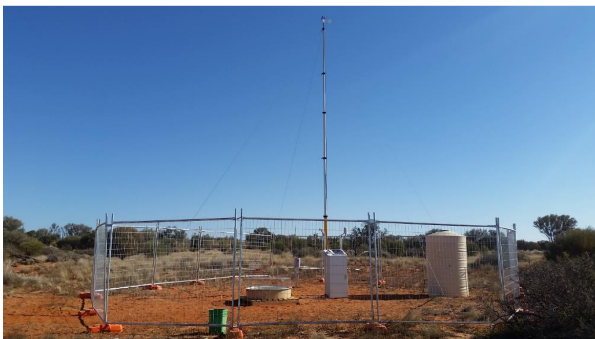
Figure 20: AWS Installed at Lake Wells
