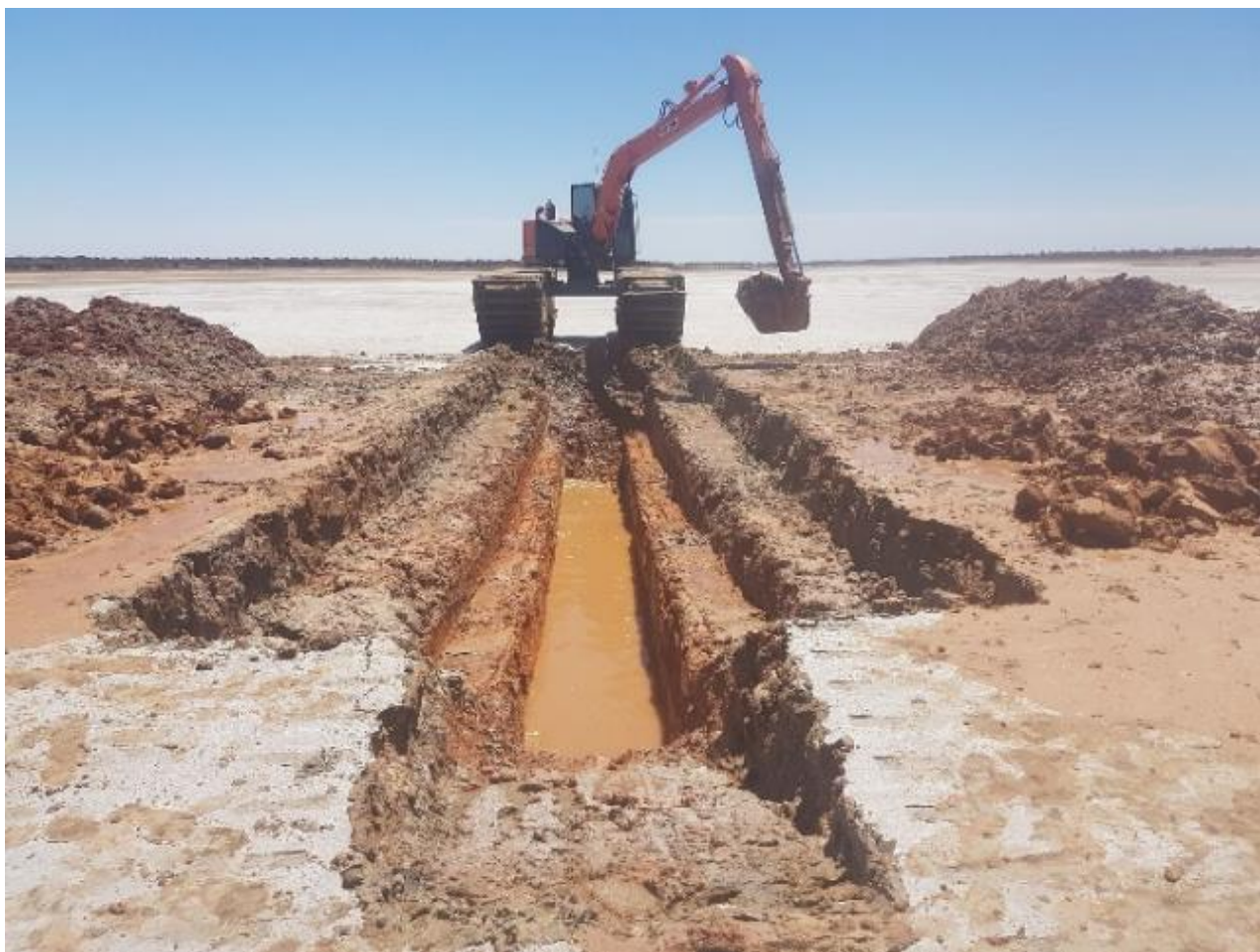
Figure 2: Test Trench Excavation at Lake Wells
