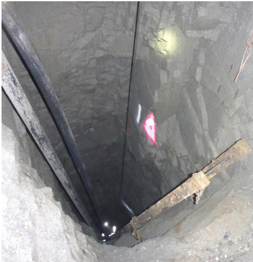
Figure 8. Air leg Egress and Escape way Rise recently completed at the A1 Mine.
