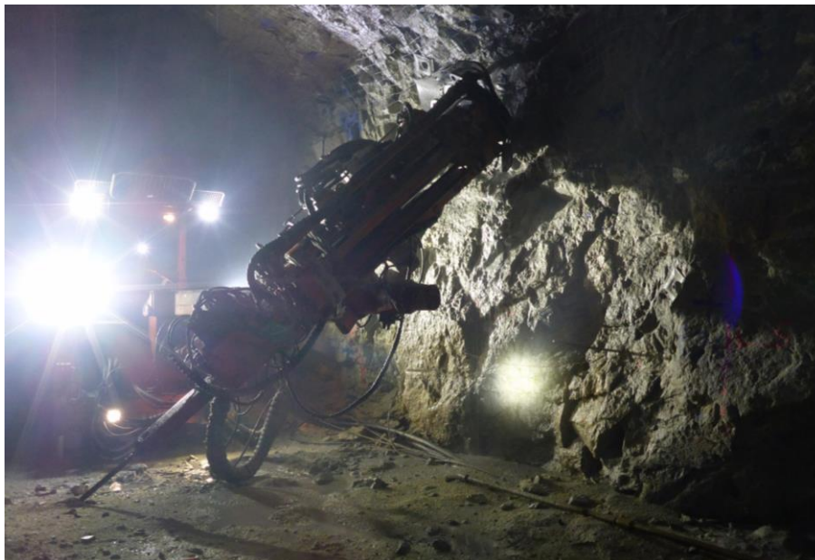
Figure 7. Long Hole Rig drilling the 1394 Long Hole Stope between 1394 to 1410 Levels.
