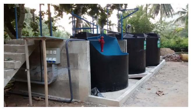
Figure 6: Shaft J mine water management & silt filtration system
