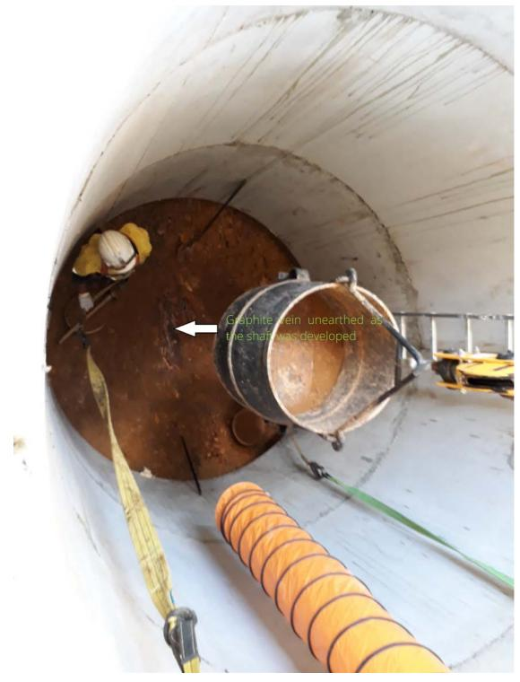
Figure 3: Shaft J 2.5 metres liner showing weathered graphite vein in shaft
