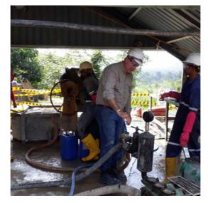
Figure 1: Managing Director, Craig McGuckin, providing instruction on pressure grouting at Shaft H
