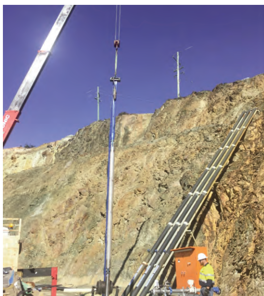
Figures 2 & 3: Installation of Woodlawn mine dewatering bore
