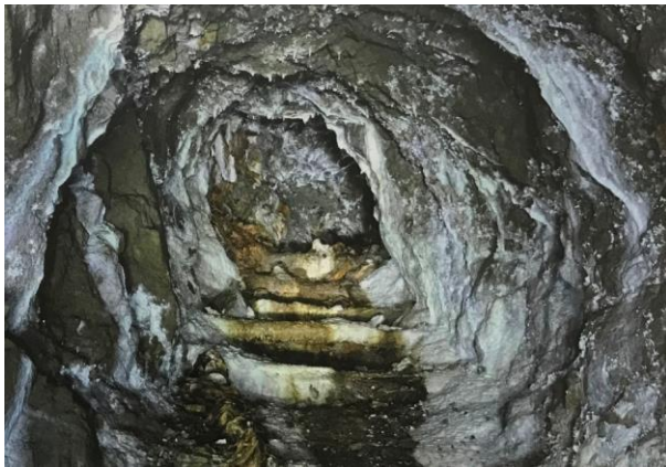
Figure 3: Gothard Underground Drive
