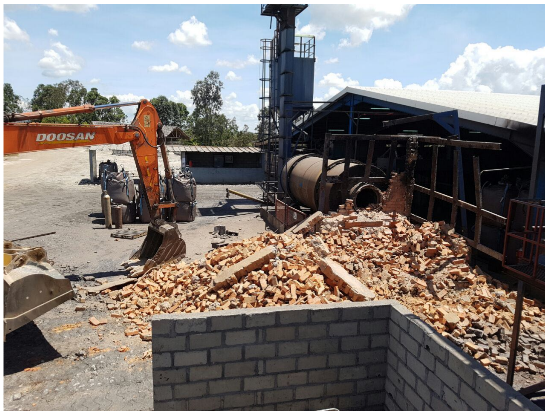
Figure 2: Rotatory drying plant de-commissioning: demolishing the brick furnace.
