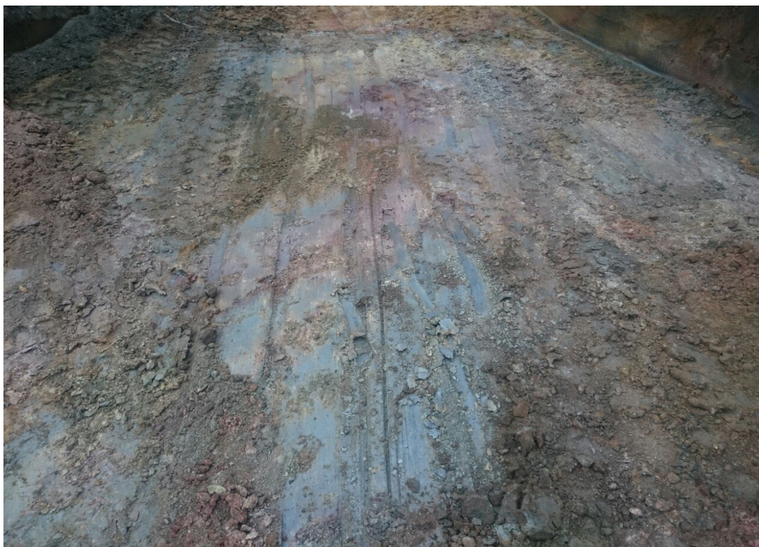
Figure 4: Mahefedok road construction uncovers soft, easily mineable graphite mineralisation (grey material) at surface.
