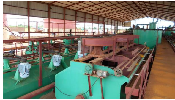
View over Flotation Circuit
