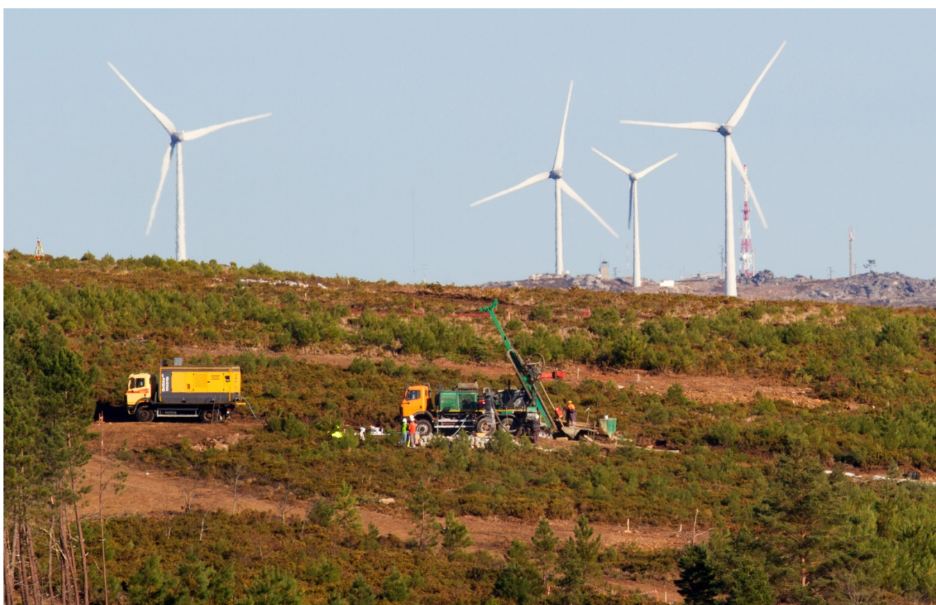
Figure 2: Drilling at Sepeda project, with wind turbines in the background.
