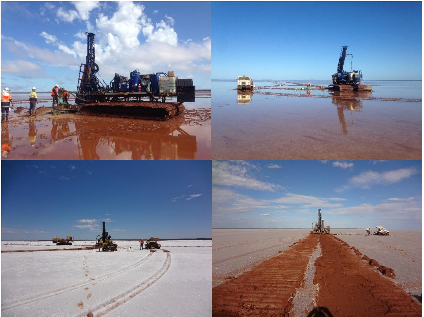
Figure 1 Examples of LEX air core drilling on Lake Lefroy February 2017
