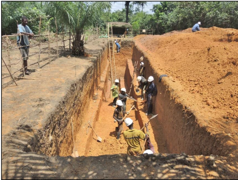
Figure 21. Excavation of trench (at left), over probe-positive KIM soil-sampling results obtained for the AM Geophysical anomaly, POD 011, EL 11/2014. The causative magnetic body proved to be a diabase dyke (at right). The source of the KIM ilmenites is unresolved.
