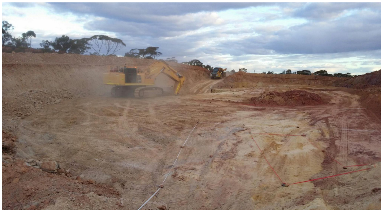
Figure 6: Boorara trial pit
