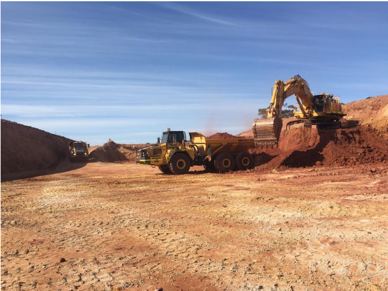
Figure 5: Boorara trial pit
