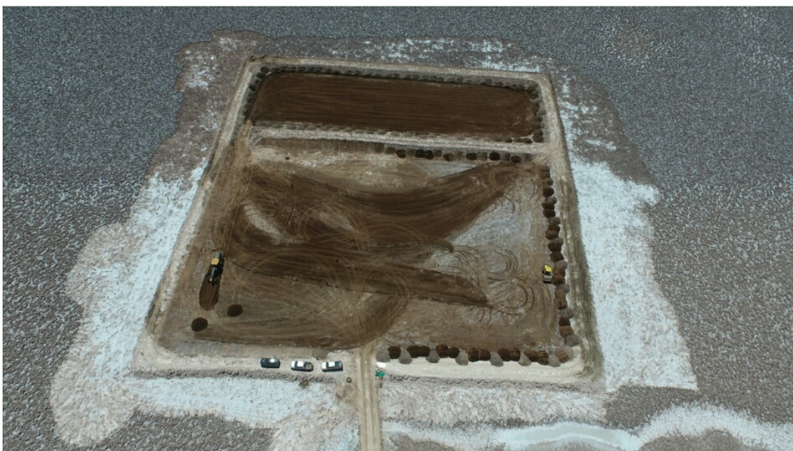
Photo 1. Rincon Lithium Project – Pond construction works.
