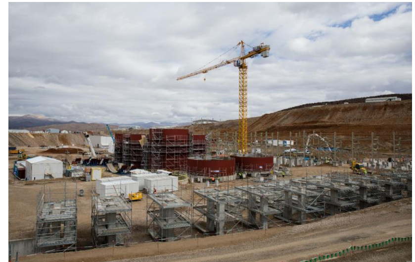
Leach and Carbon-in-Pulp Tanks
