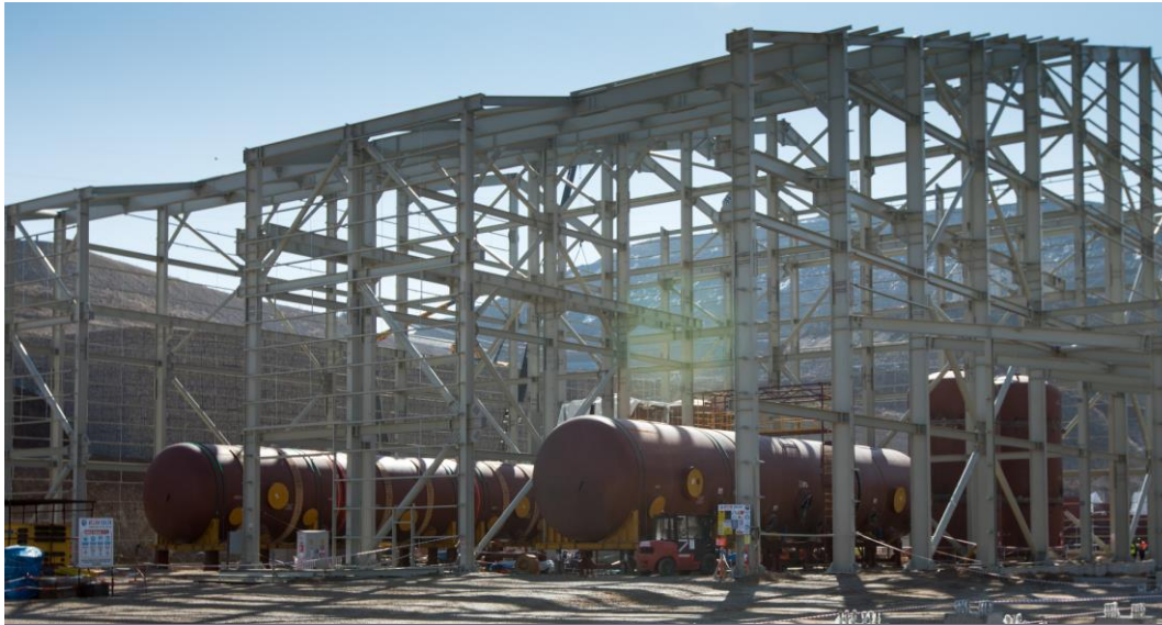
Autoclaves in Pressure Oxidation Building
