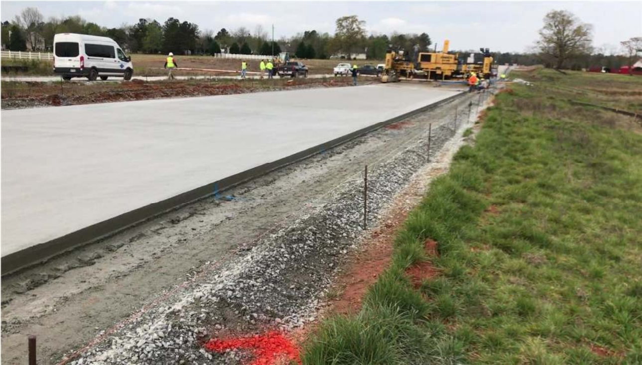
Figure 2. Completed section of highway with added EdenCrete®
