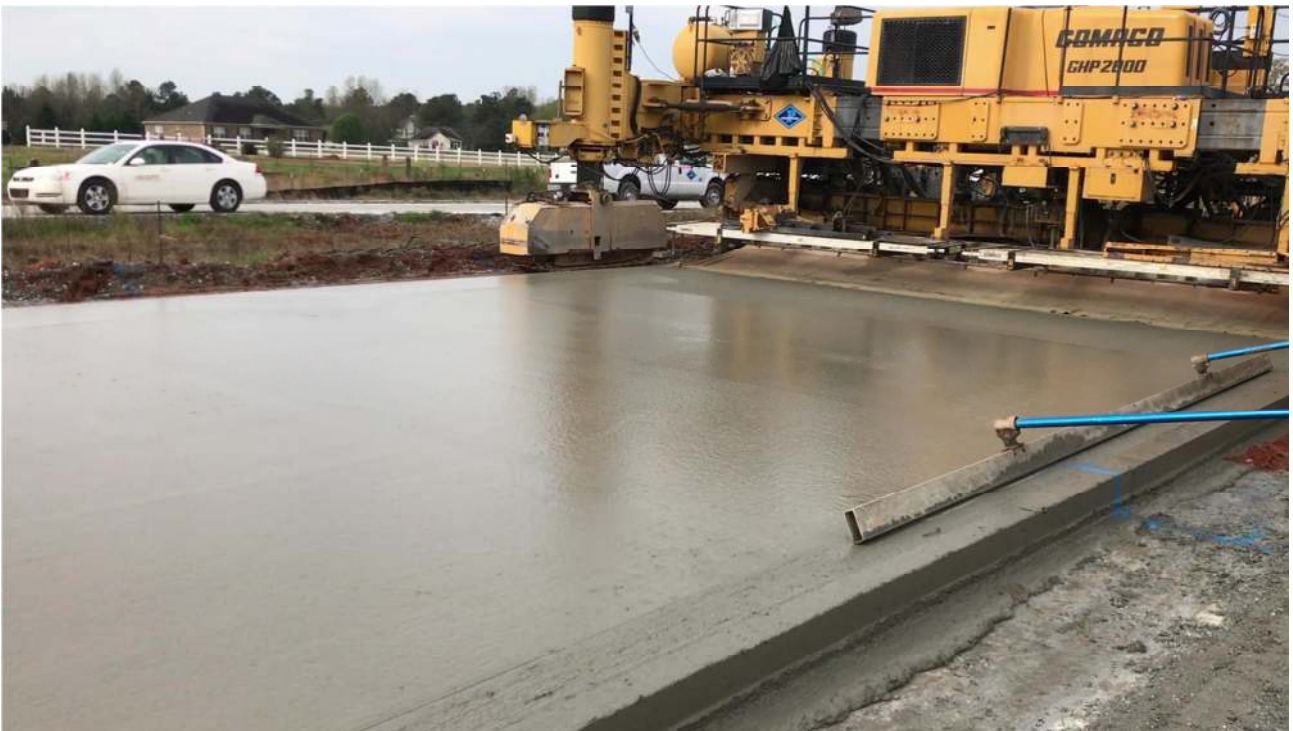
Figure 1. EdenCrete ® - enriched concrete being laid in Field Trial
