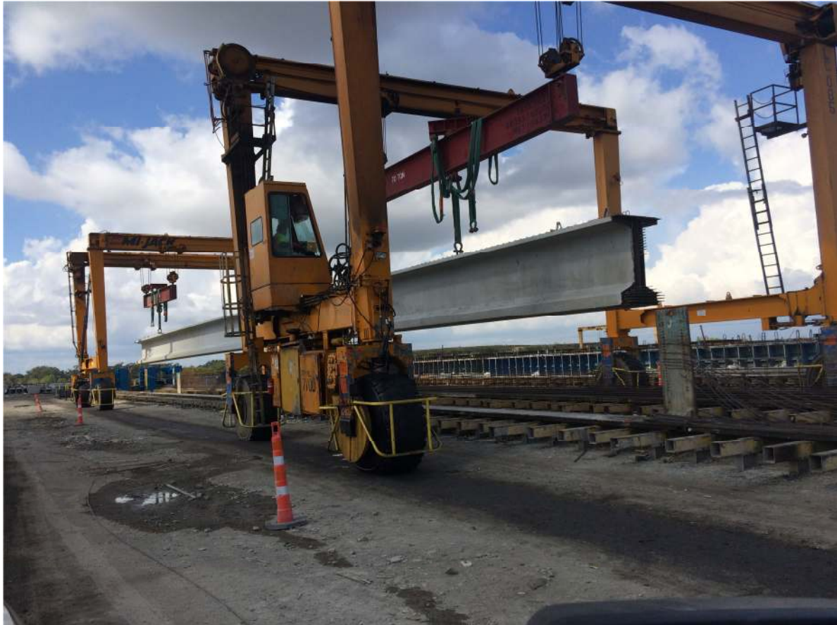
Figure 1. Typical prestressed bridge beam being fabricated
