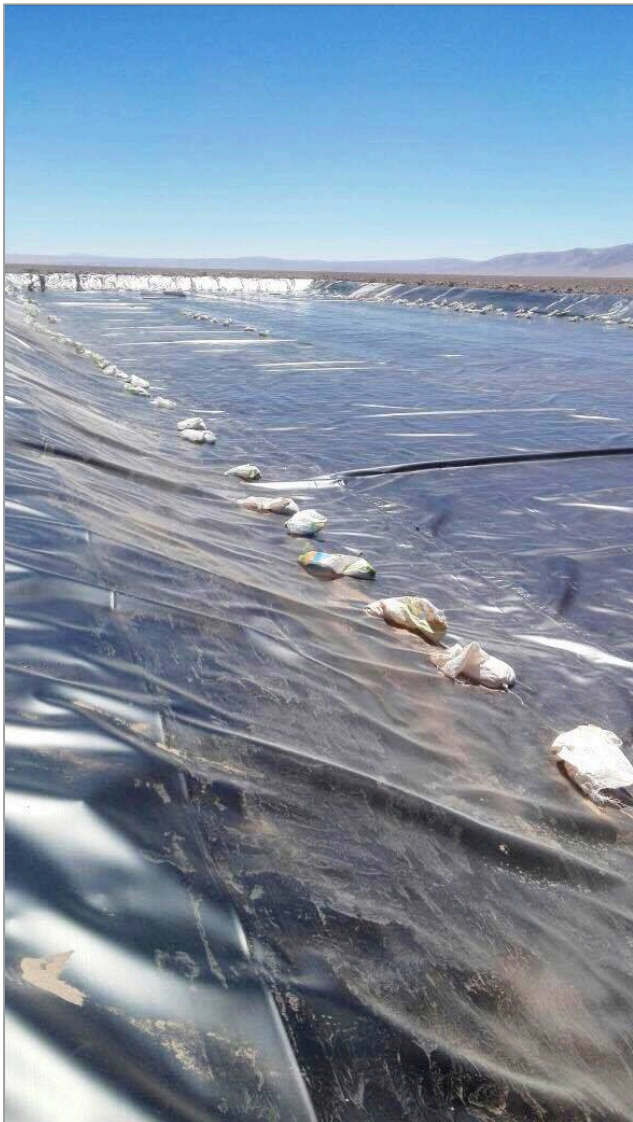
Photo 1. Rincon Lithium Project – Pond construction works; lining installation of Pond 2.
