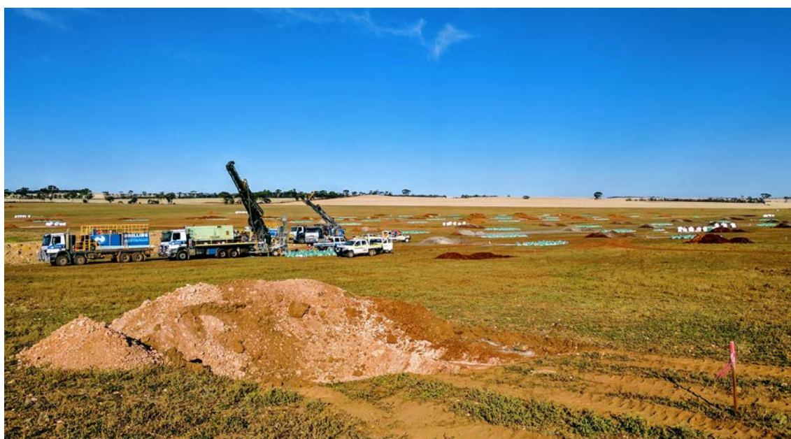
Drilling the Leicester gold zone at Tampia
