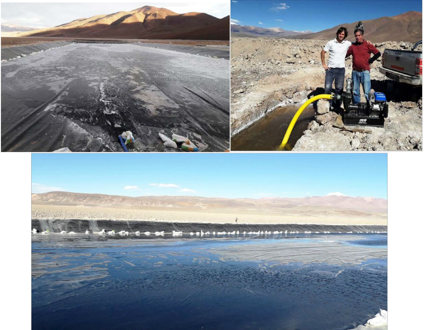
Photos 1 - 3. Rincon Lithium Project – First brine in ponds.
