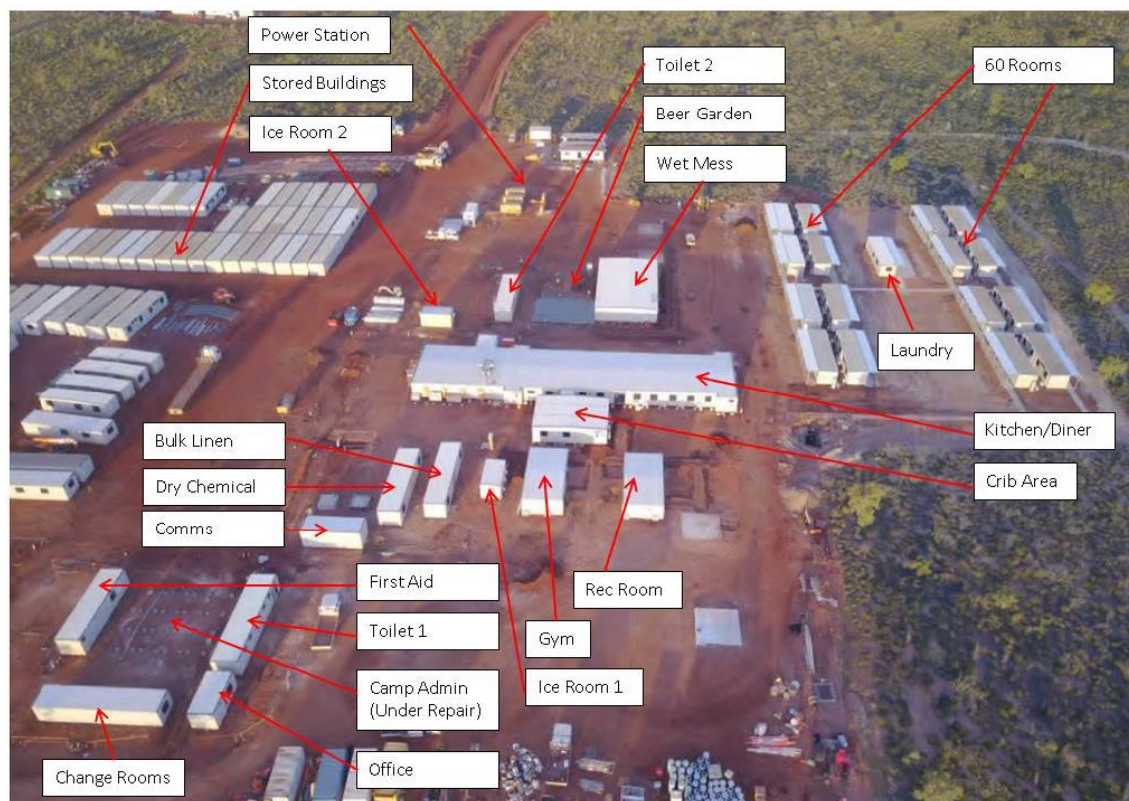
Figure 4 – Camp Development, with final installation of first 60 rooms (to right of photo)
