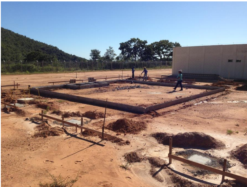
Figure 2: Laboratory civil works as at 10 April 2017
