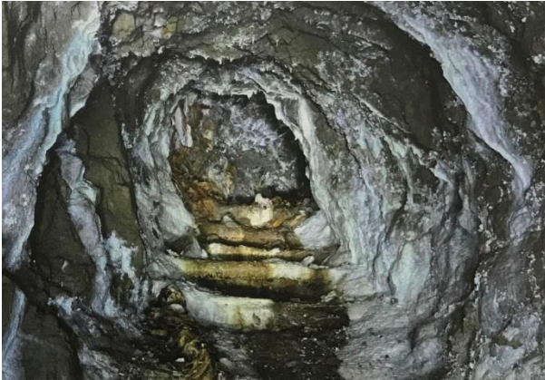
Figure 3: Gothard Underground Drive
