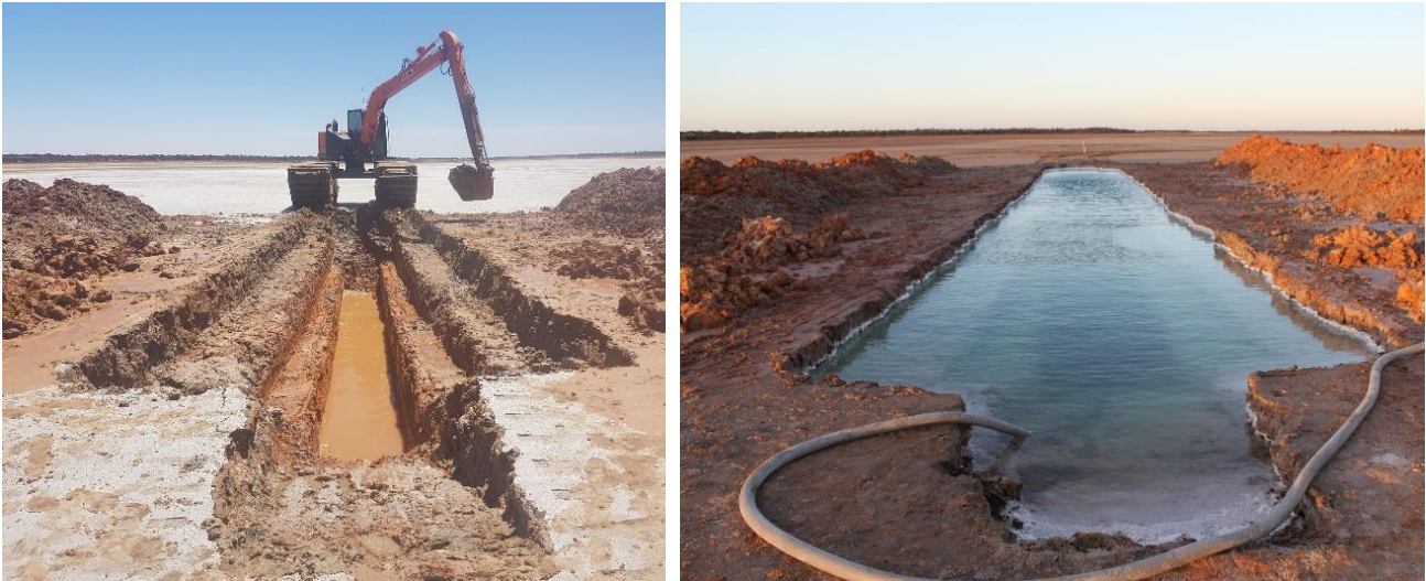
Figure 2: Test Trench Excavation and Trench Pumping at Lake Wells
