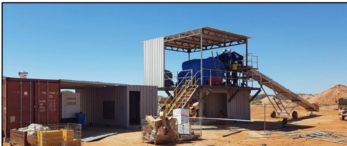
Figure 1: Ore Sorting Module under constrction (including compressor station – insert)
