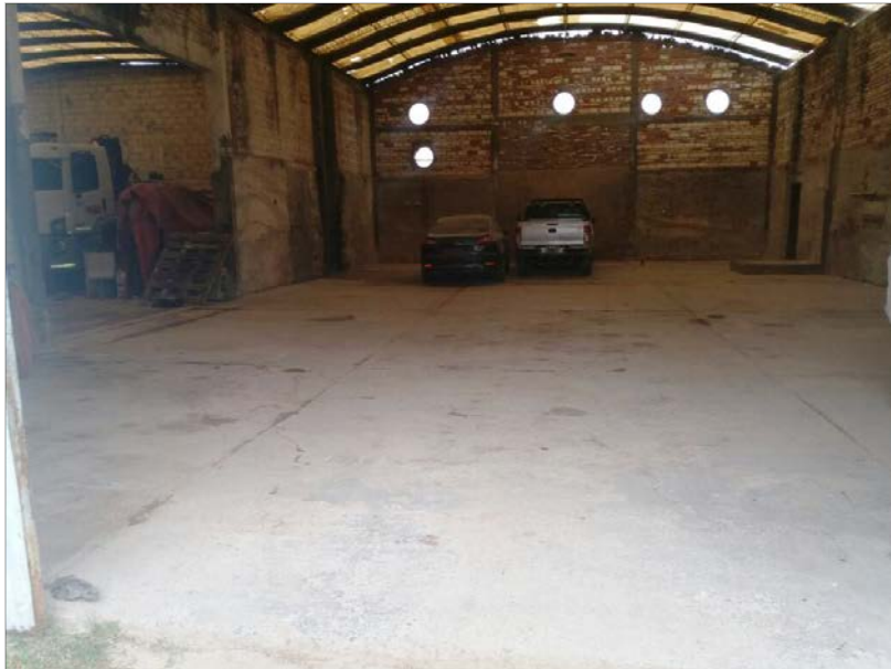
Photo 4. Rincon Lithium Project – Warehouse at industrial site.
