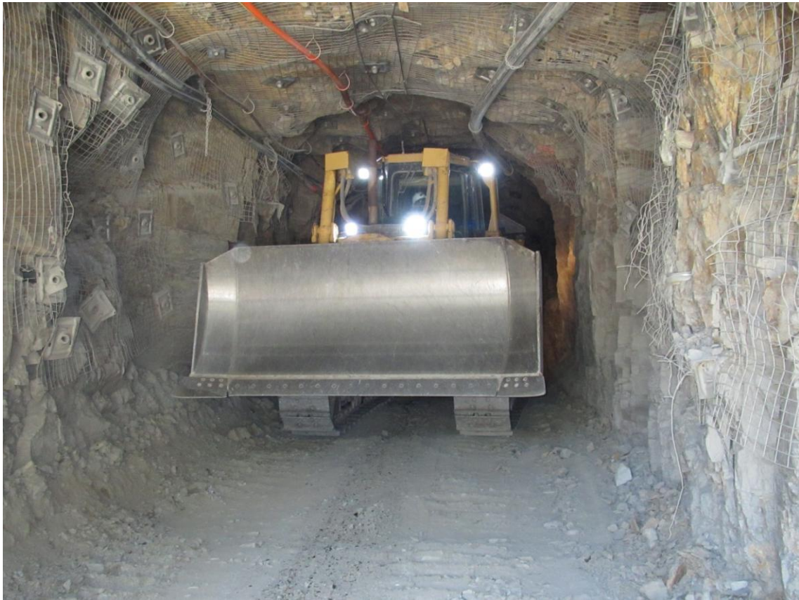
Figure 1. Photo of dozer ripping the decline at the A1 Mine
