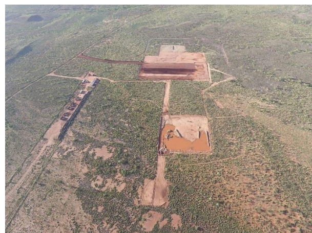
Figures 8 & 9 – Camp Site Bulk Earthworks and Temporary Offices
