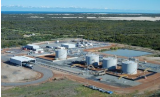
Photo: Arrowsmith Stabilisation Facility
