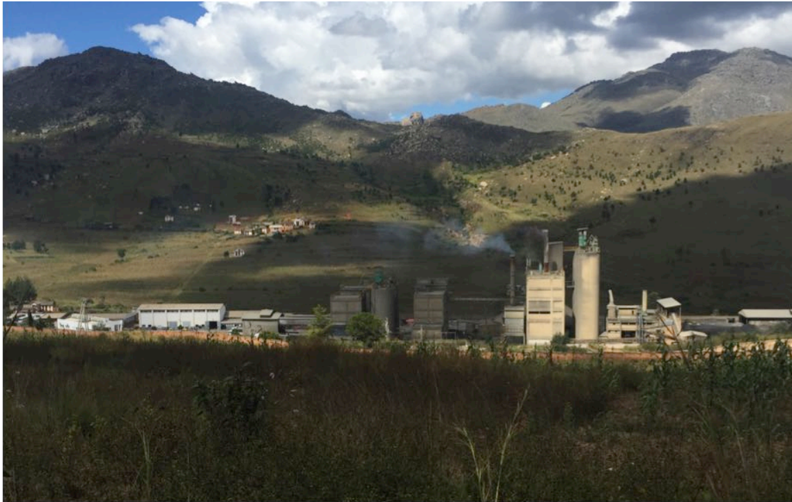
Figure 3: Holcim's talc processing facility with grid power, adjacent to Millie's Reward.
