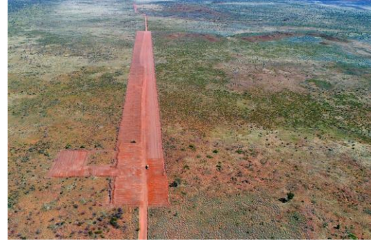
Browns Range Airstrip – topsoil cleared
