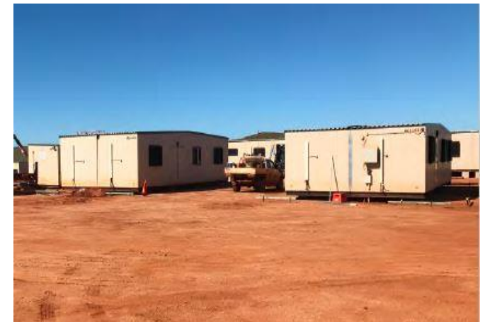
CAMP BUILDING INSTALLATION
