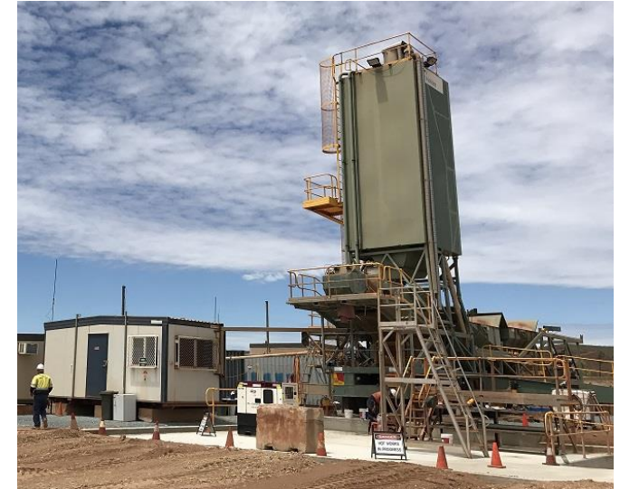
CONCRETE BATCHING FACILITY
