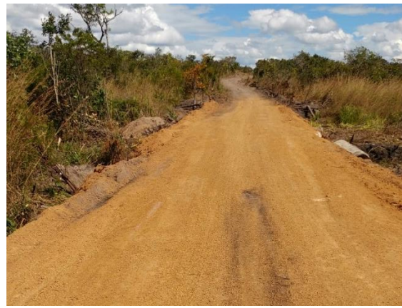
River Crossing 1 (after)
