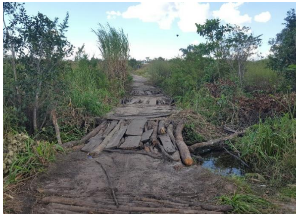
River crossing 1 (before)
