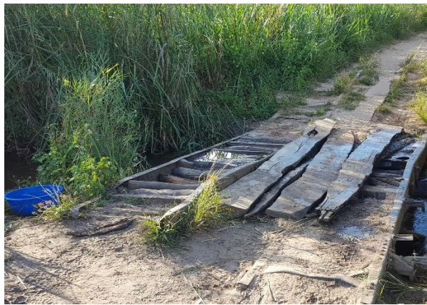
River crossing 2 (before)
