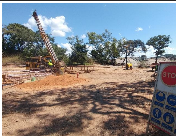
Geotechnical Diamond Drilling at Kalongwe Pit
