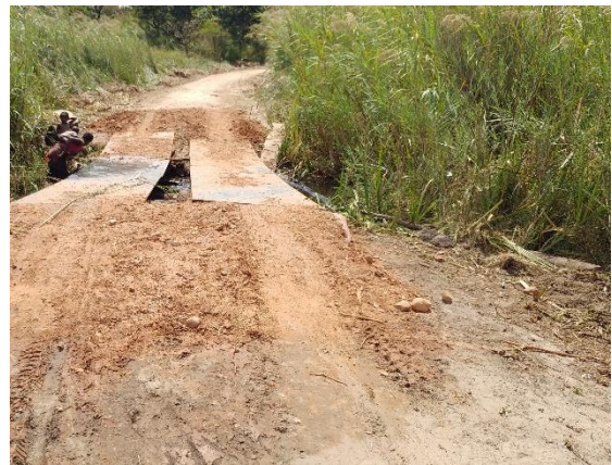
River Crossing 2 (after)
