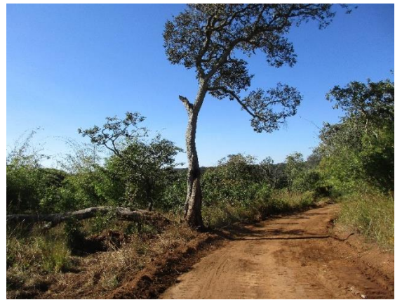
New 36km access track (after)
