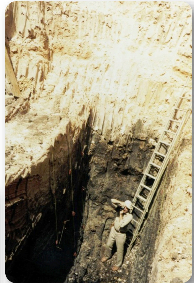
Close-up in Japanese test pit (1980s) showing carbon-rich ore and free dig nature of material
