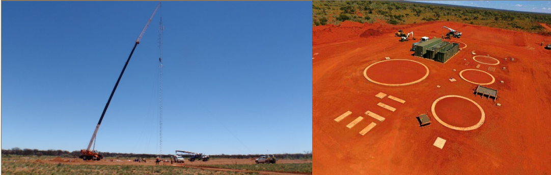
Construction of infrastructure underway
