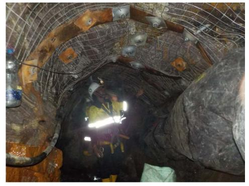
Note extensive rock bolting and meshing in Shaft H, drive H036196
