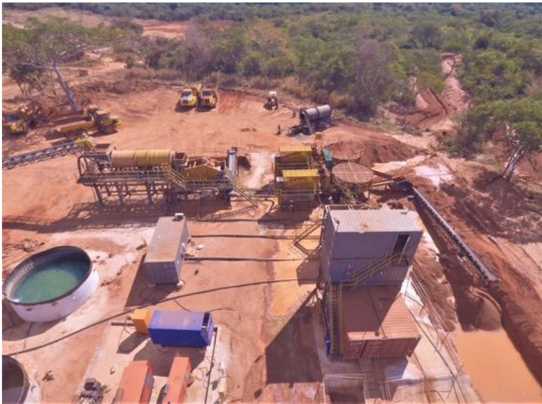
Figure 1. Newly upgraded 250tph processing plant in operation
