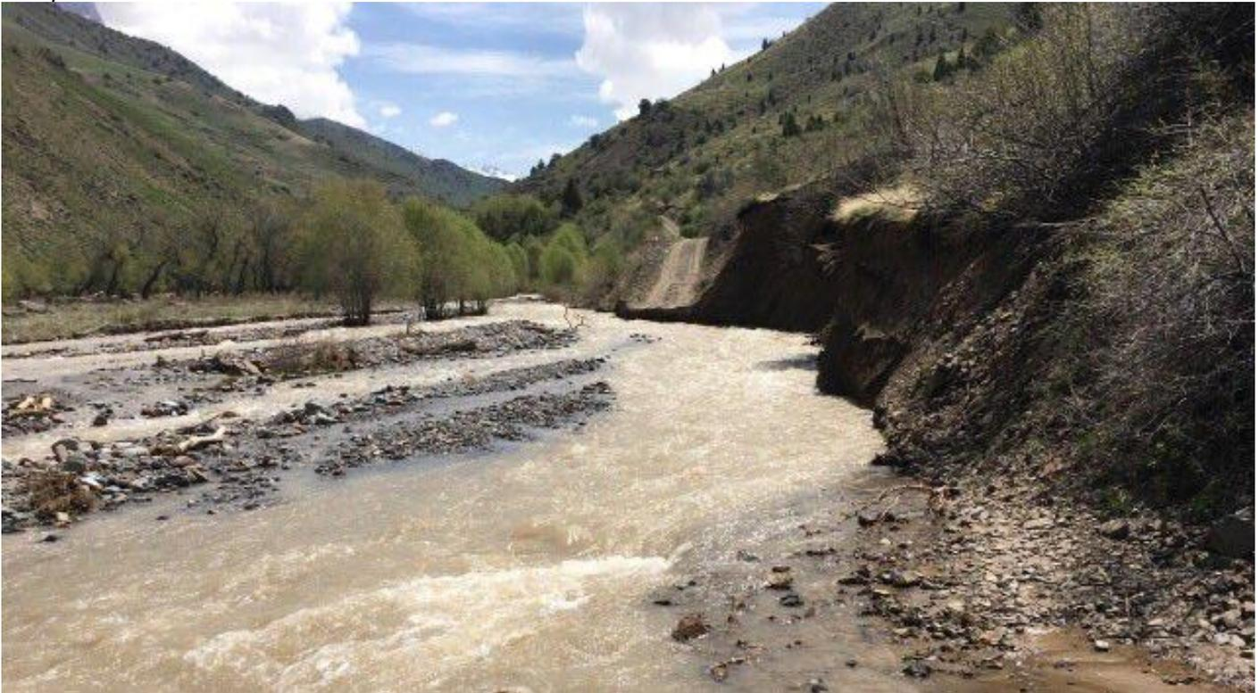
**Figure 6:** Snowmelt water scouring river crossing track along the Chanach River.
