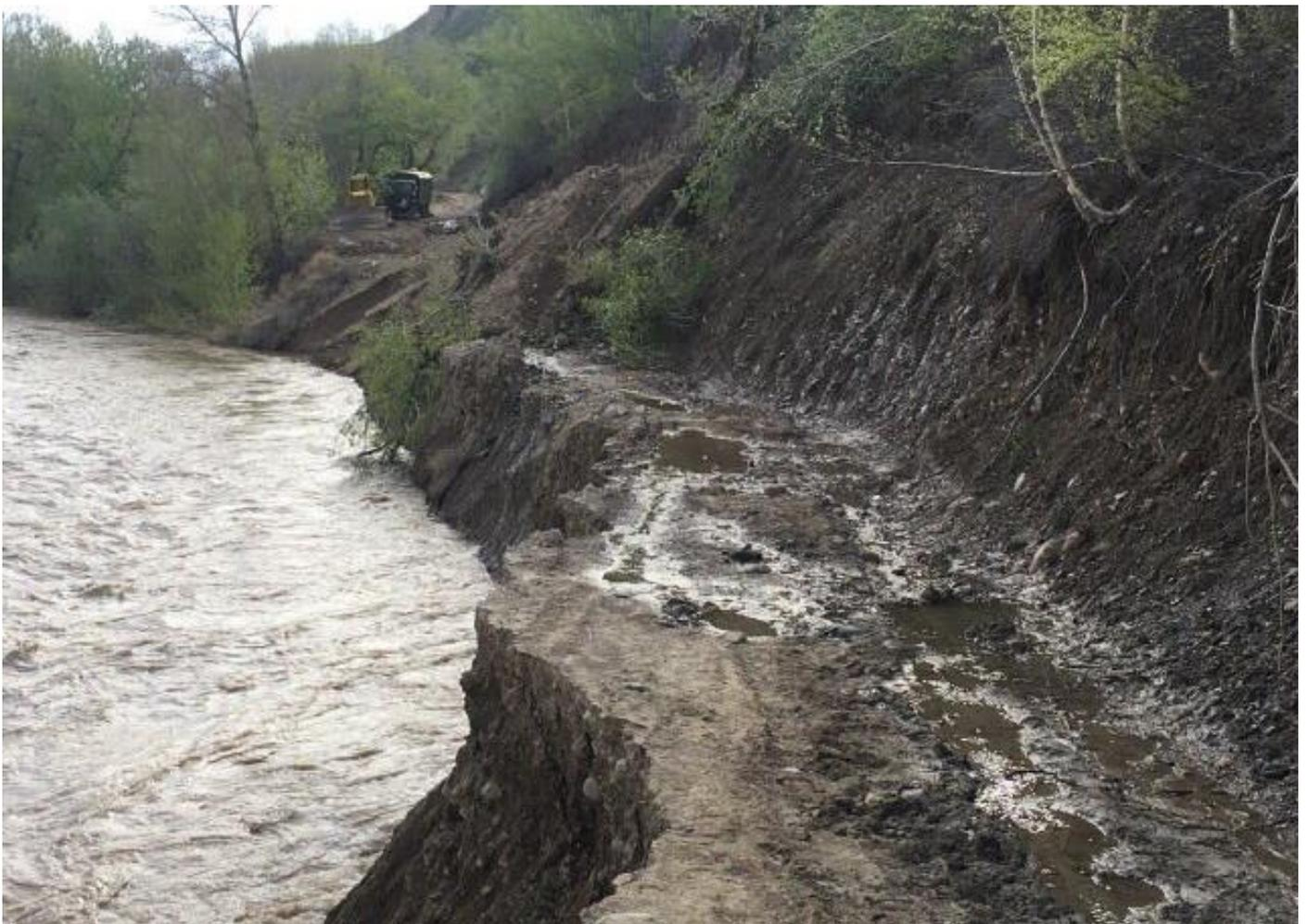
**Figure 3:** Access road in main Chatkal valley washed away by the Chatkal River. An alternative access track has been established.
