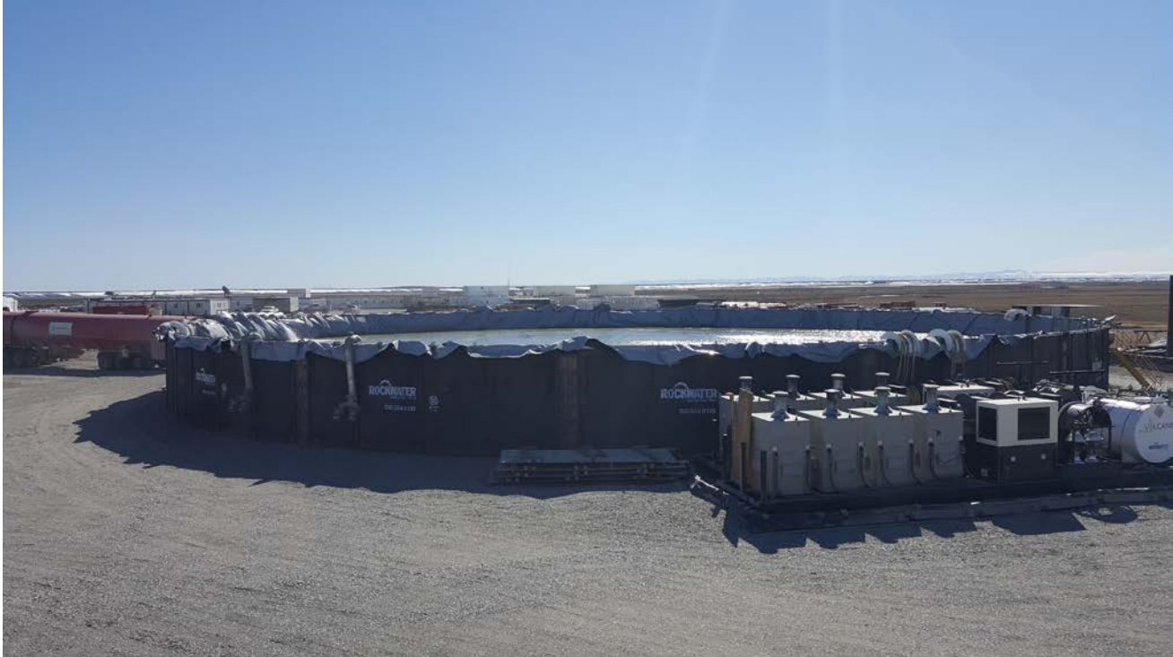
Fig.1 Stimulation Water Reservoir on Location at Franklin Bluffs
