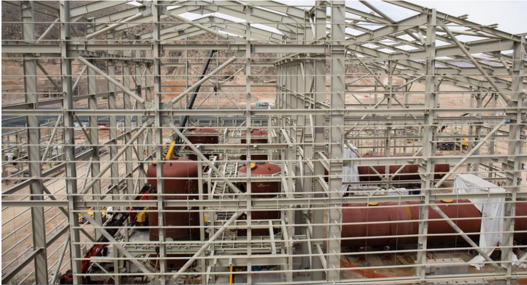
Autoclave Building with Flash and Autoclave Vessels in Position
