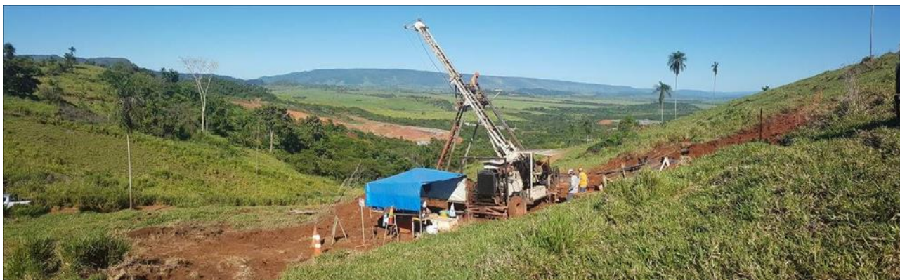
Figure 1: Drill hole AAND-100 in progress, with the Antas pit in the background
